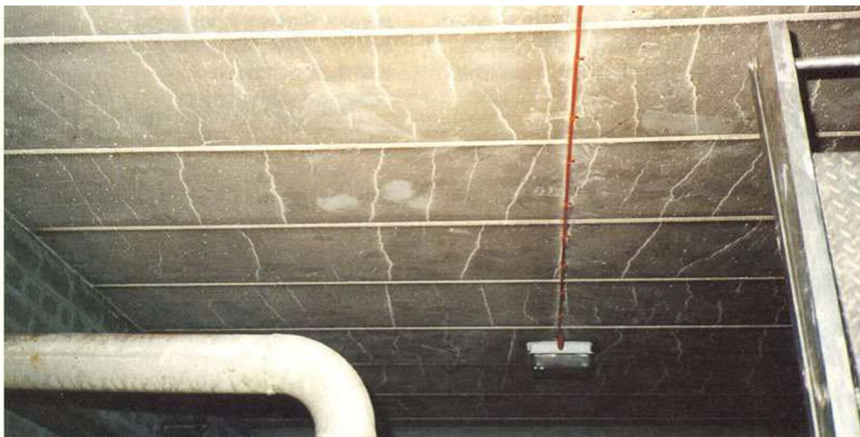
**Figure 2** Widespread hair-line cracking on the soffits of many RAAC planks
